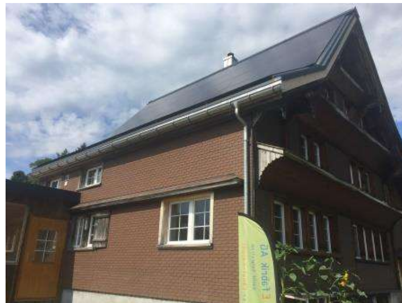
EFH Ebnat-Kappel 11 kWp Indachmontage
